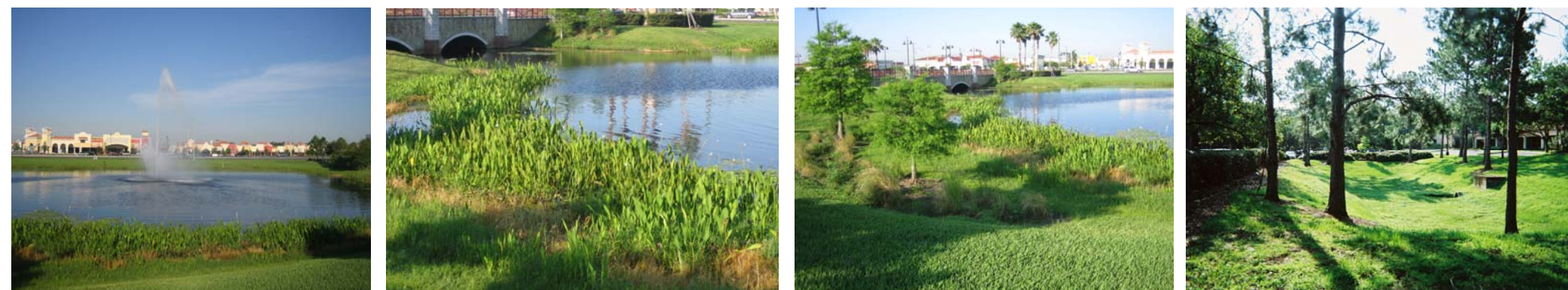
Figure 14: Wet and Dry Retention Ponds
