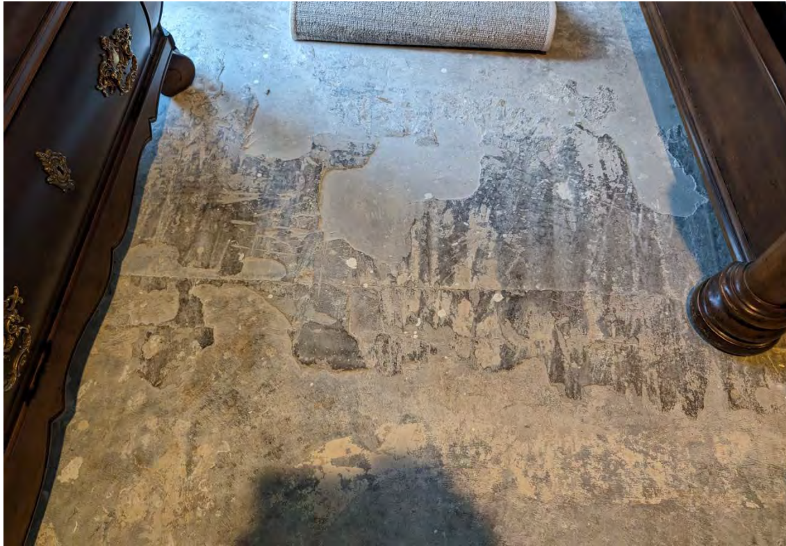
Concrete Slab Tie-in, Master Bedroom Addition
