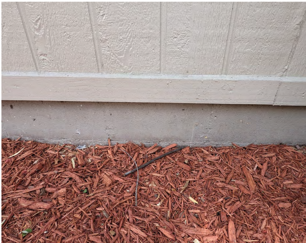
Stem Wall on Strip Footing
